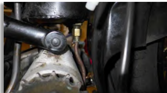
Figure 24: The vent pipe of the oil tank can now be unscrewed.
